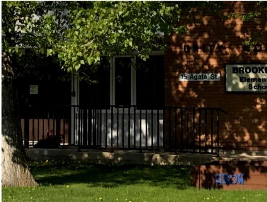
Brookdale School - Front Entrance
